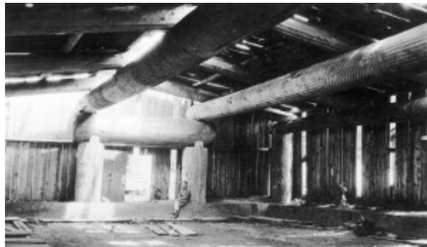
Figure 13.3 Despite efforts to rehouse Aboriginal people in Euro-Canadian structures, longhouses were still be built in the 20th century. This one is under construction in the Vancouver area around 1912.
