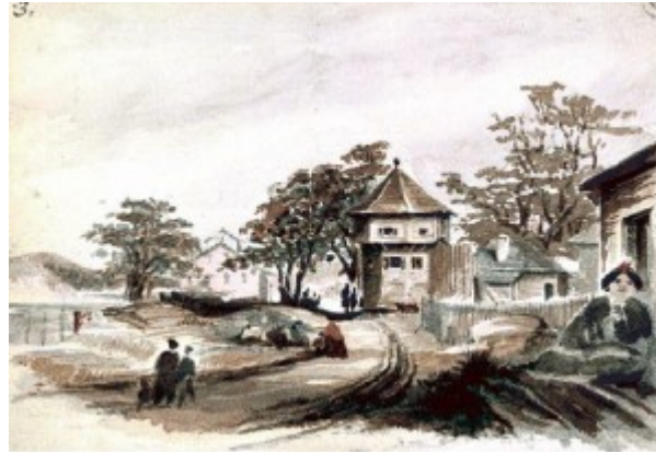
Figure 13.24 The southwest bastion of the HBC fort at Victoria, 1860. (Watercolour by Sarah Crease.)
