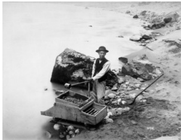
Figure 13.31 Chinese miners introduced machinery like this “rocker” on the Fraser River ca. 1875.
