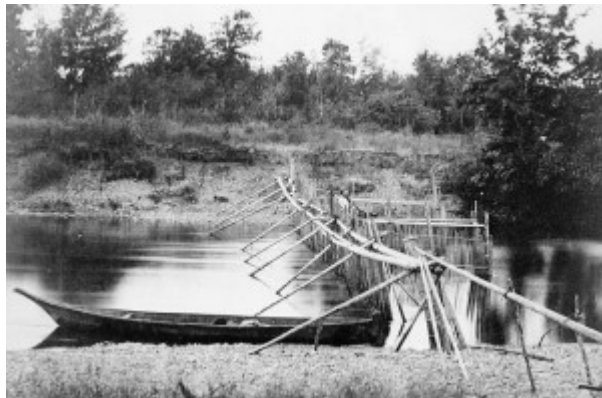
Figure 1.9 Fishing weirs like this one from the Cowichan River (ca. 1866) were built by Aboriginal peoples across Canada long before contact. Wood, a readily available building material in northern North America, was used far more widely than stone, but it leaves less evidence behind.
